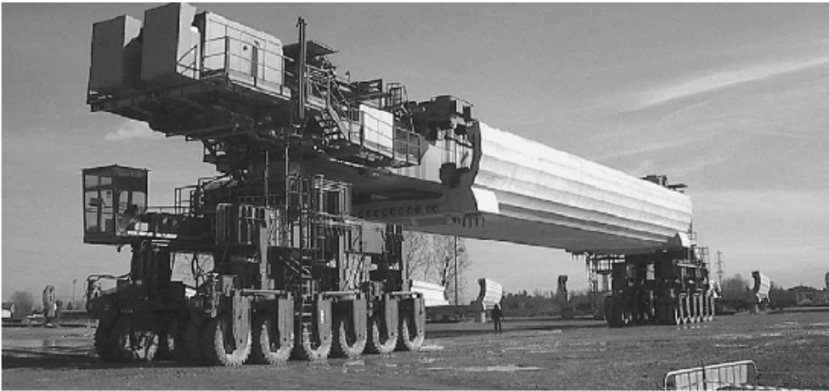
Modena precast deck lifted and transported on tyres from stocking area, Milano-Bologna line.
